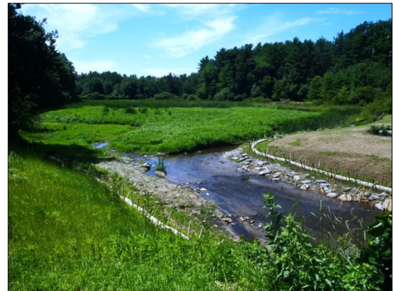
Dam removal complete
