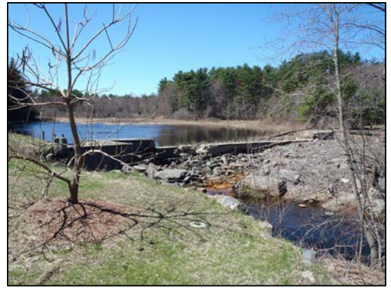
Dam prior to removal
