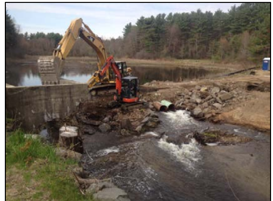
Dam removal in progress
